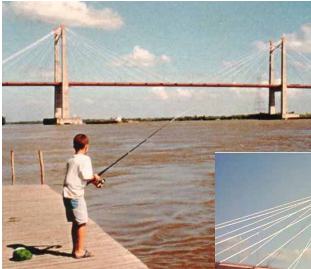
Zarate-Brazo Largo, 1978.g, 2003.g, Argentina 110 m + 330 m + 110 m H piona = 110.00 m h grede = 2.60 m
