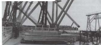
Fig. 7.63 Prefabricated truss elements for the sway bracings and the vertical main trusses of the Akashi Kaikyo Bridge after having been lifted onto the bridge deck at the pylons
